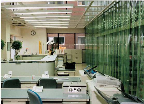
事務所の省エネに For saving energy in office
